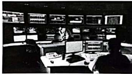
Command and control center
