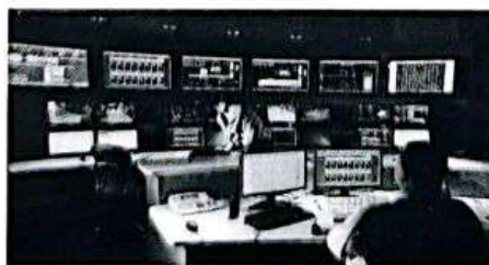
command and control center
